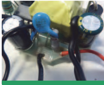
Fig 5 Point at which Sample No. 6 failed the electric strength test
